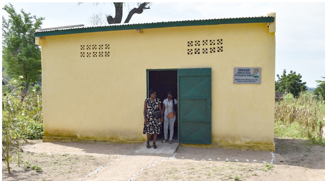
Storage shed built
